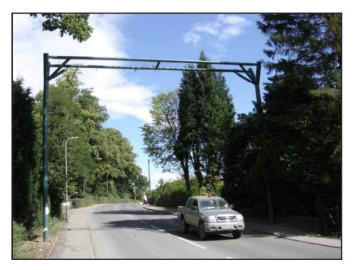
Figure 6. Bat crossing at Sirhowy.
