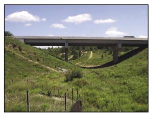
Figure 15. Landform Conservation-Three-span 81-meter Bridge
