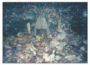
Figure 7. Main causes of misfunctioning amphibian mitigation measures I.: lack of maintenance (Henley-on-Thames, England).
