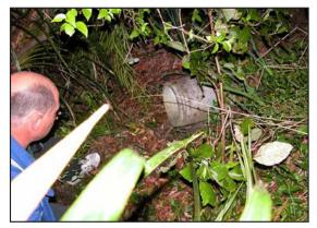
Figure 8. Main causes of misfunctioning amphibian mitigation measures II.: construction problems (tunnel entrance over the ground), besides the fence is lacking (near Auckland, New Zealand). (Photo courtesy: Dr. Phil J. Bishop)
