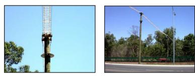
Figure 11. 60m-long rope ladder-style arboreal overpass erected in open forest habitat in Brisbane, Queensland. (Photos by Pauline Fitzgibbon)
