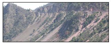
Figure 1. Disposal of cut material downhill into the Alaknanda River caused by the widening activities on NH-58.
