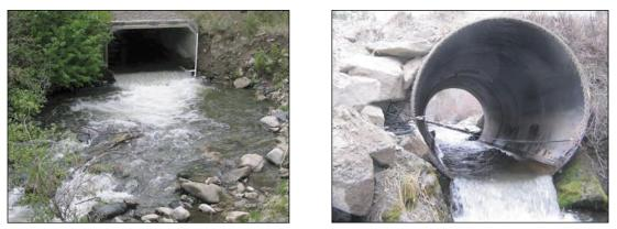
Figure 2A. The outlet of culvert 1, a box pipe (I), and the outlet of culvert 4 (r).
