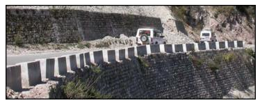
Figure 6. Early failure of toe wall due to heavy precipitation during monsoon (July-August) on NH-58.
