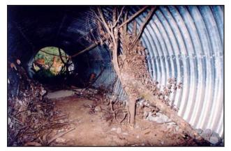
Figure 2. Faunal underpass showing furniture, including escape pole (vertical tree branch), sand bed, attractive habitat at exit, soil, litter, rocks and logs to simulate rainforest floor conditions.
