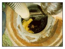
Figure 3. Vacuum truck employed during the cleaning operation of a water-quality inlet along the Southeast Expressway in Boston (left) and a maintenance worker pushing sediments to a vacuum hose while exercising "confined-space entry" protocol (right).
