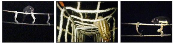
Figure 9. Ringtail possums using arboreal overpasses: left and right – Lemuroid and Herbert River ringtail possums on 14-m-span rope ladder over a sealed tourist road; center – Green ringtail possum in a rope tunnel over 7-m-wide unsealed road clearing.
