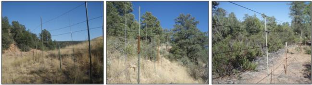
Figure 2. Applications of modified right-of way fence raised to 2.2–2.4 m to funnel wildlife to underpasses, a bridge, and the animal-activated detection system crosswalk, including fence raised with: 1) 3-m T-posts and barbed-wire (left), 2) T-post sleeve extensions and barbed-wire (middle), and 3) ElectroBraid™ braided rope electric fence and fiberglass posts (right).
