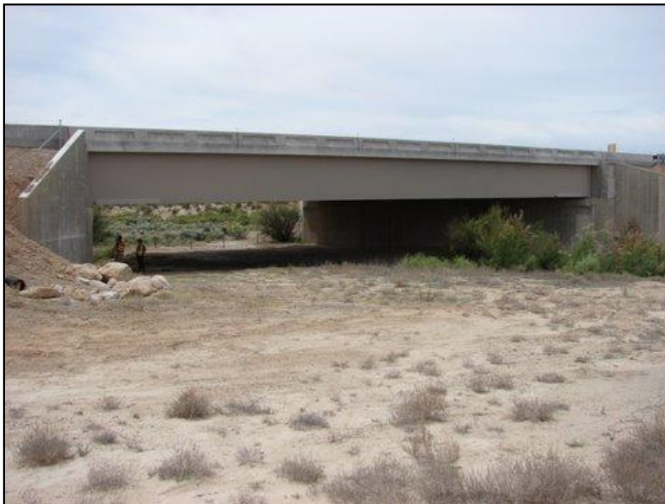
Photo 3. Large bridge across Grassy Trail Creek, US 6, Utah. This existing bridge is larger than would likely be built for a wildlife crossing. It is suitable for antelope, mule deer, desert carnivores and other small animals. It is also in a stream channel that wildlife often use for travel and dispersal. Photo by Ruediger.
