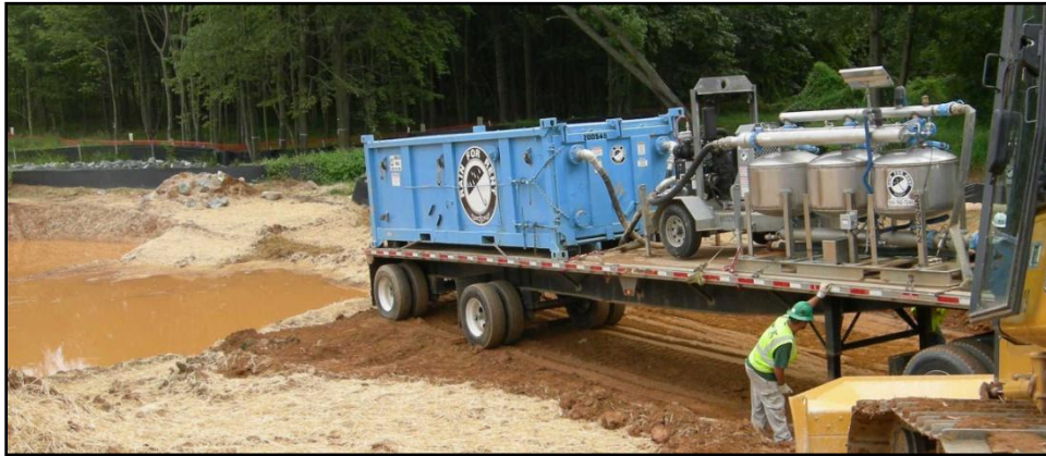
Figure 7 - Rain for Rent® Unit Using Flocculents
