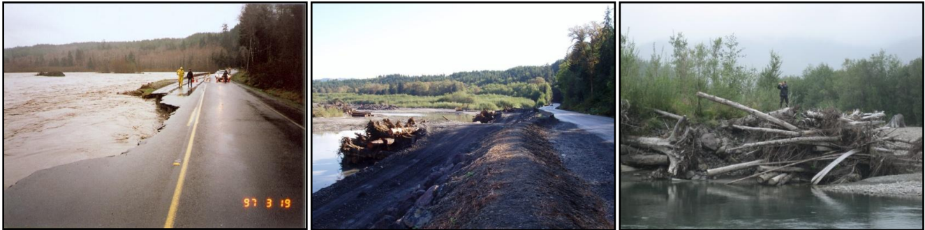
Figure 3: Damage to US 101 adjacent the Hoh River, left, resulted in one of the first CED projects including bank stabilization structures, center, and large mid-channel ELJ's, right.
