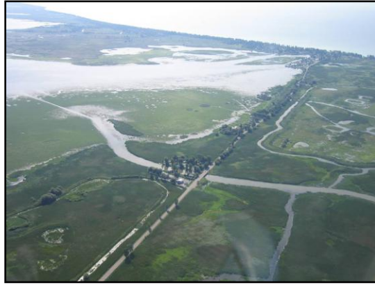
Figure 4. Big Creek outlet under causeway, with impoundment area in right central part of photo and Lake Erie at top of photo (Photo courtesy of Scott Gillingwater).
