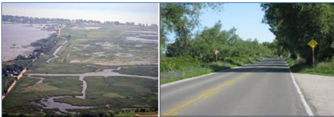
Figure 2. Causeway Setting. Photos: Ecoplans Limited (2007/2008).
