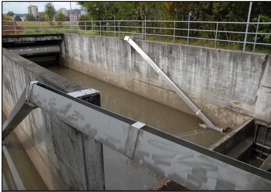
Figure 8. Installation of ramps in every rain retention basins.
