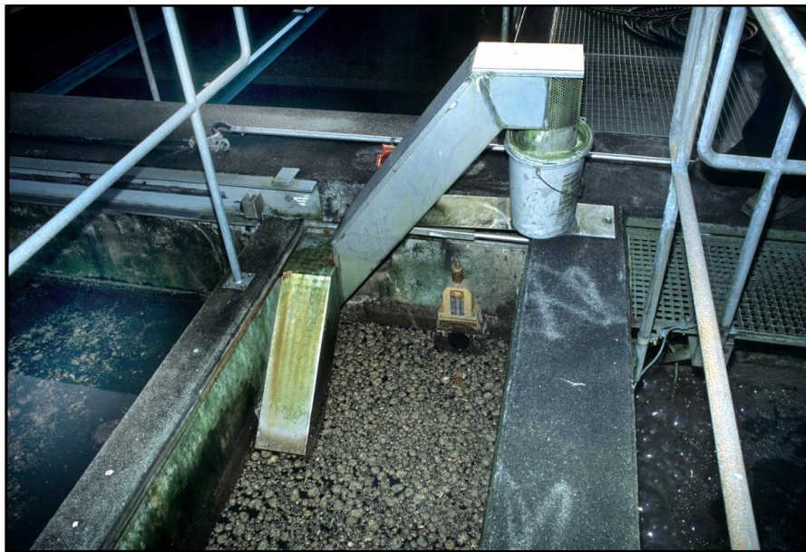
Figure 9. Lack of space obliged the construction of a steep ramp with 60° and a 90° curve, a protection against the sun is necessary.
