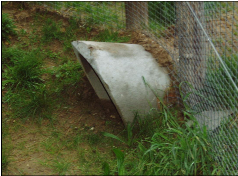
Figure 2. New badger tunnel.
