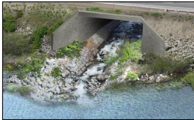
Figure 10. A conceptual four-sided box culvert design for Wolfe Creek
