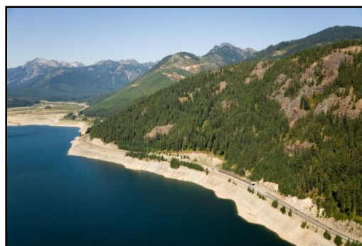
Figure 2. The I-90 Hyak to Keechelus Dam project corridor. This section of I-90 rests between Keechelus Lake and steep cliffs
