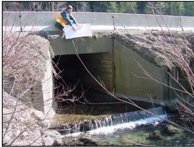
Figure 9. The existing Wolfe Creek 6-foot box culvert
