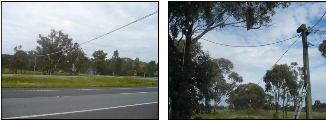
Figure 1. Canopy bridge spanning dual-carriage Hume Highway, Victoria. Photo on right shows “feeder” ropes, connecting the end of the canopy bridge to adjacent trees.
