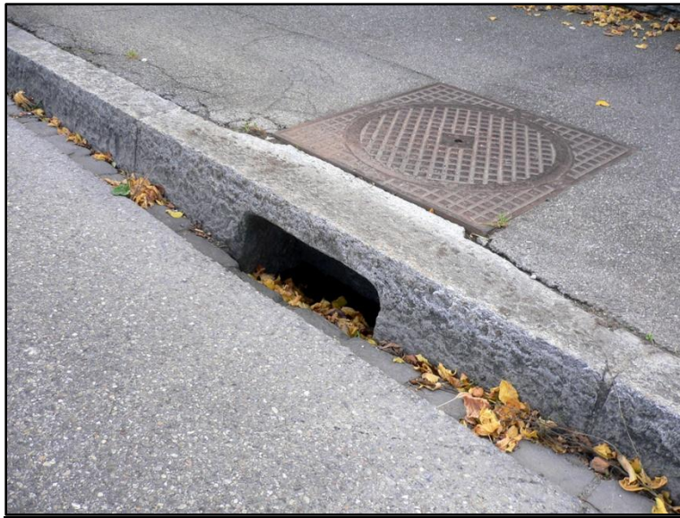
Figure 1. The gutter leads small animals to this curb inlet.
