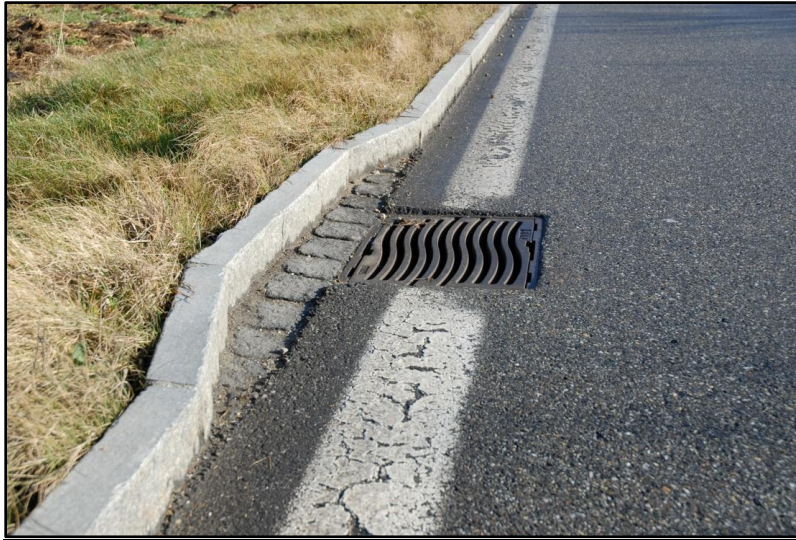
Figure 2. Amphibian friendly storm drain: By setting the curb back so as to permit animals to bypass the drain. In this case the gridding is also narrower, which avoids animals from falling in.
