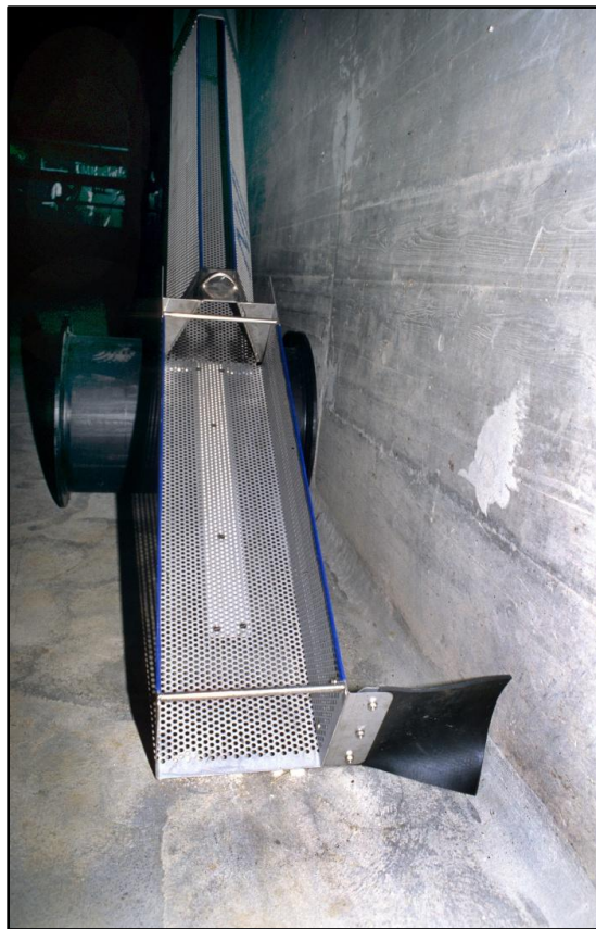
Figure 6. To help the animals find the ramp it is important that no space is left between the wall and the escape platform. In this example, the space is closed with a rubber flapper.
