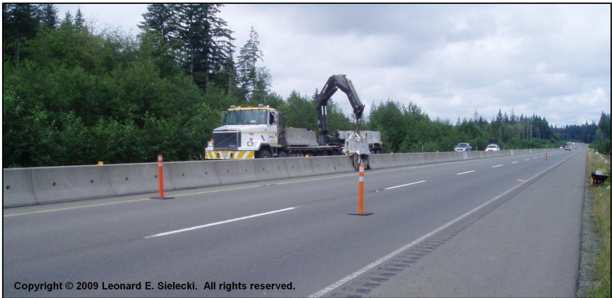
Figure 6. Lane Closures and Installation of Scuppered Concrete Median Barriers
