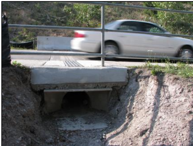
Figure 4. Completed tunnel under the Entrance Road. Tunnel mouths were later covered with biodegradable matting to stabilize soils and provide more natural cover. Photo courtesy of Parks Canada.
