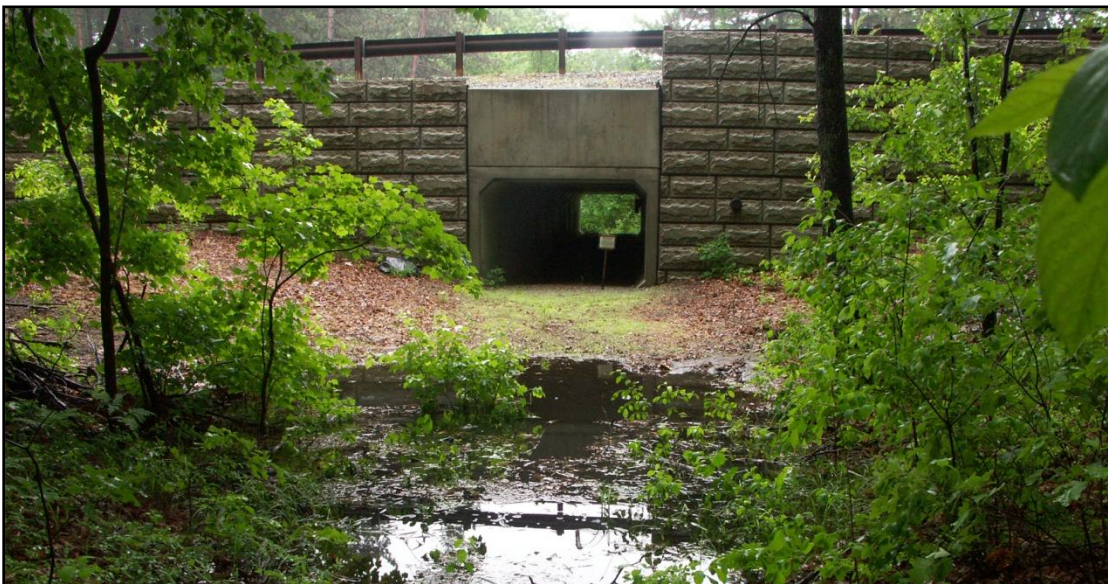
Figure 3. Photograph of underpass # 1
