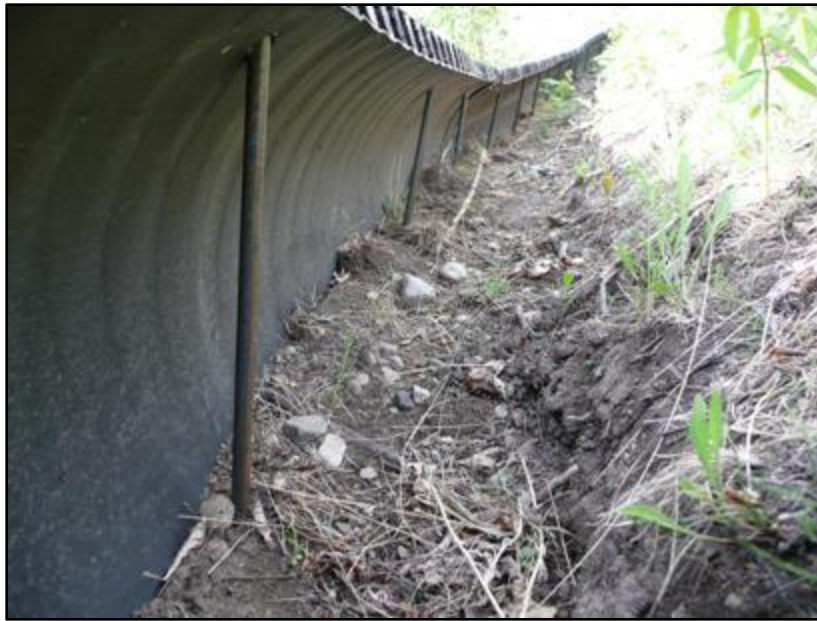
Figure 5. Ground-level view of section of HDPE plastic pipe. Photo courtesy of Parks Canada.
