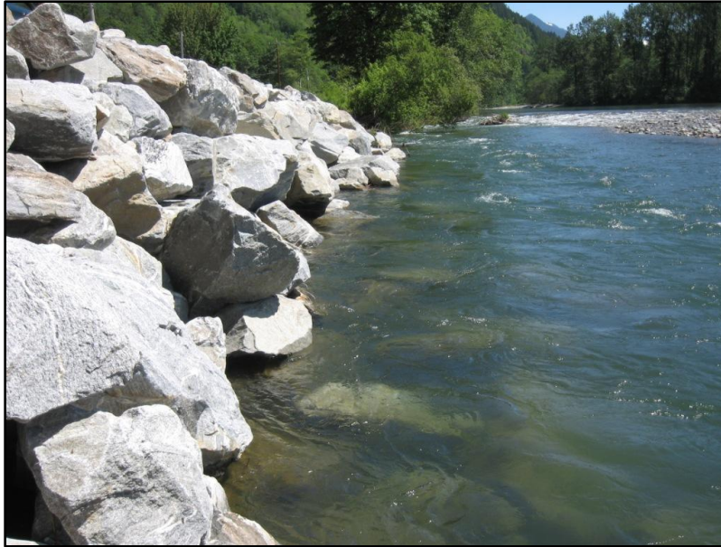
Figure 1: A usual approach to protecting road infrastructure is placing large rip-rap, such as this temporary revetment along SR20 on the Skagit River.
