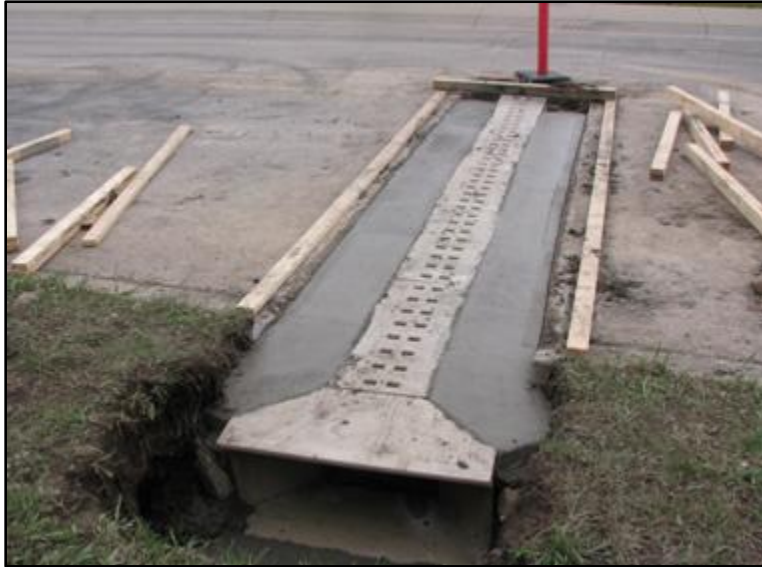
Figure 3. Half of one tunnel waiting for concrete to set, before diverting traffic and completing second half of tunnel. Photo courtesy of Parks Canada.
