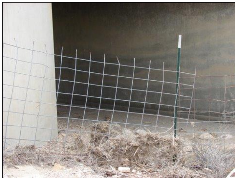
Figure 4. Example of welded livestock panel blocking two large box culverts on Icelander Creek, US 6, Utah. These culverts would be used by large and small wildlife if livestock fencing were modified and wildlife wing fences installed. Photo by Ruediger.
