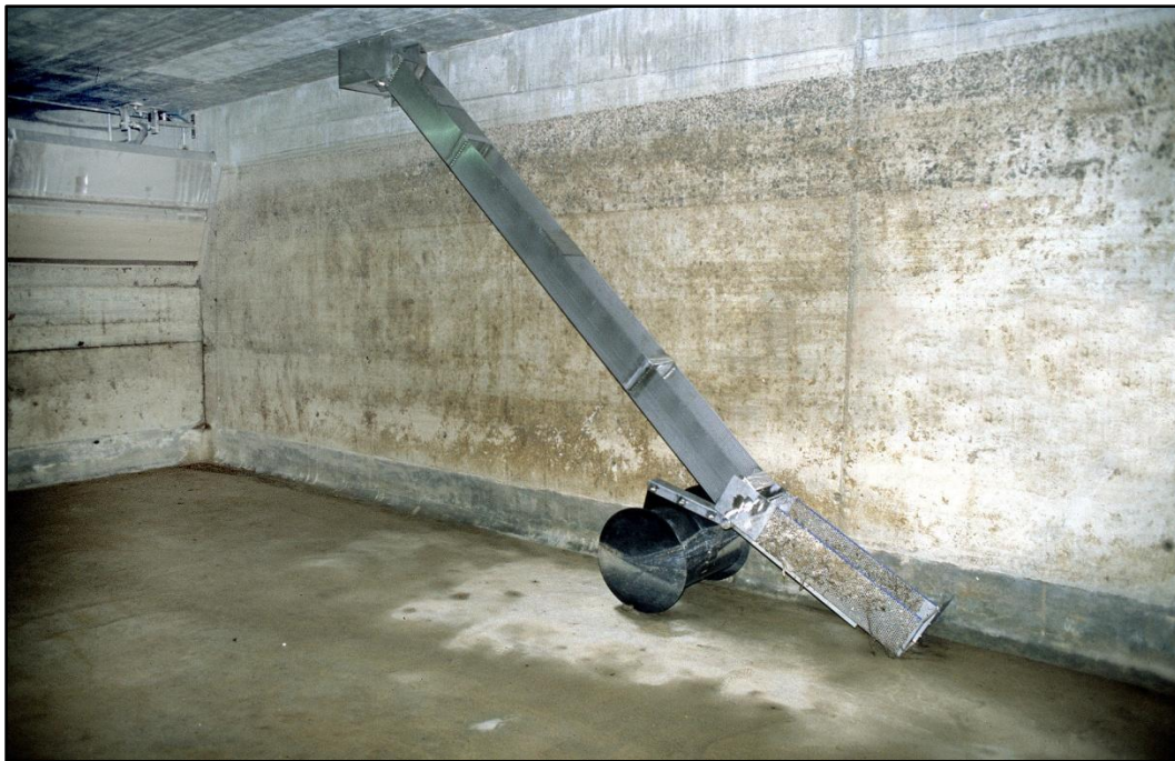
Figure 4. Example of an escape ramp from an underground storm water tank.
