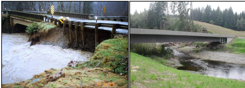
Figure 4: The old US101 bridge over Nolan Creek, left, was a safety hazard and constricting the creek. The CED program replaced the bridge with a clear span bridge to allow channel migration, right.
