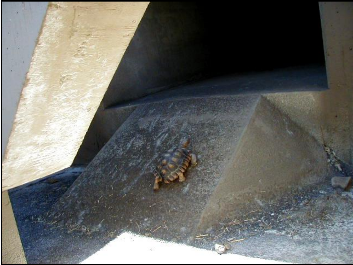
Figure 3. Desert Tortoise Going up Incline to enter Culvert (Photo by ADOT/USDA Forest Service).
