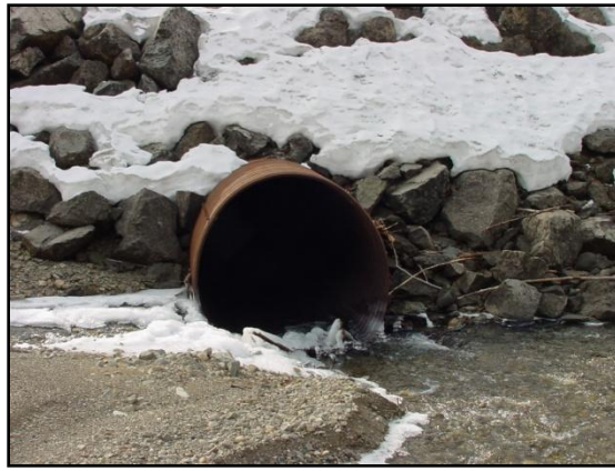
Figure 12. The existing 6-foot pipe culvert at Resort Creek
