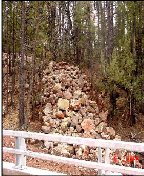
Figure 1. Elk Riprap (Photo by ADOT).
