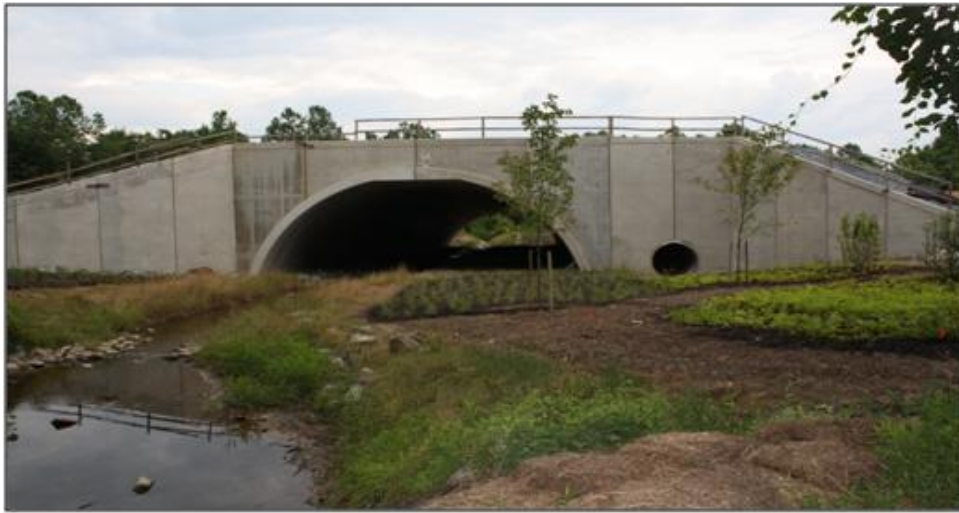
Figure 8 - Culvert Z: Bio-Sensitive Bottomless Arch Culvert
