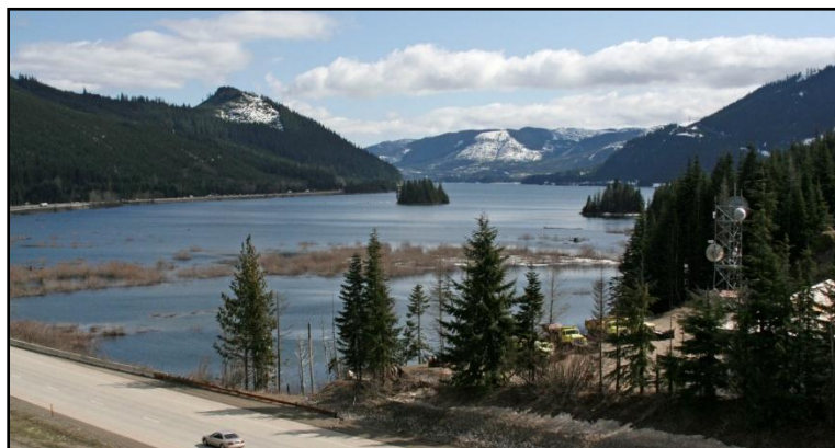
Figure 7. I-90 (lower left), Keechelus Lake (center), and the WSDOT Maintenance Facility (lower right). The facility provided a suitable stormwater treatment / snow storage area
