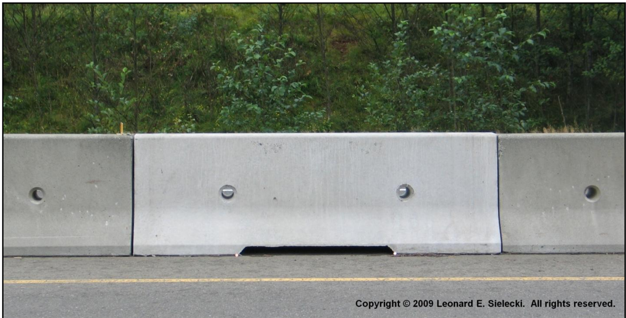
Figure 7. Installed Scuppered Concrete Median Barrier
