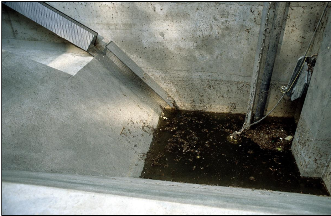
Figure 5. The escape platform must reach to the sump pit. In narrow systems it is important that design takes such aspects in account early in planning.
