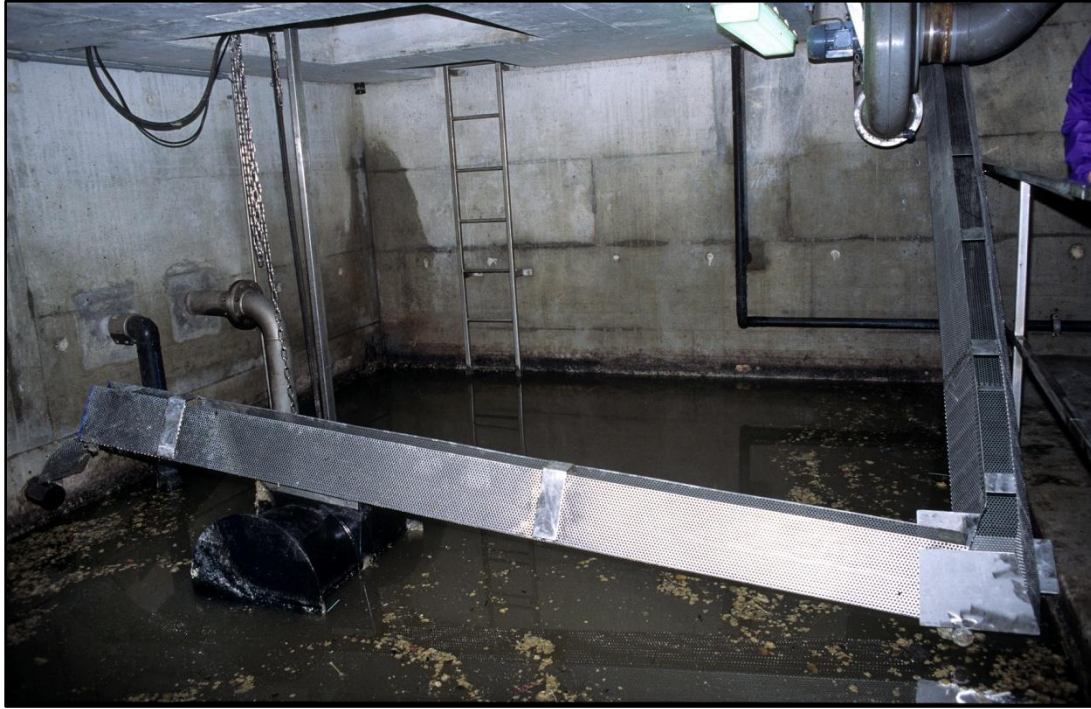
Figure 10. Installation of ramps in an underground pumping station with narrow dimensions.
