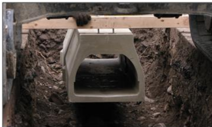
Figure 2. Tunnel segment, suspended flush with surface of pavement, above trench to be filled with concrete. Photo courtesy of Parks Canada.
