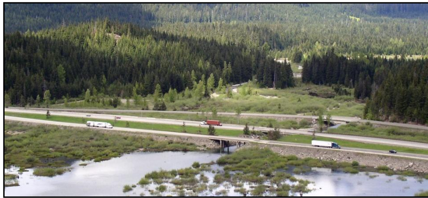
Figure 3. The existing Gold Creek Bridge
