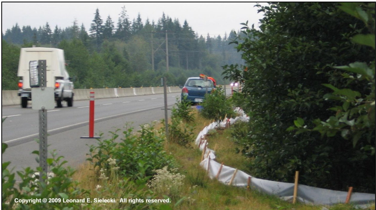
Figure 8. Temporary Amphibian Fencing in Highway Right-of-Way
