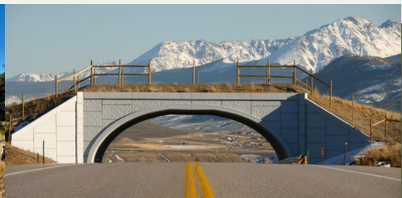
CO 9 Wildlife Overpass
