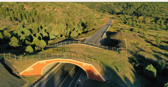
US 160 Wildlife Overpass
